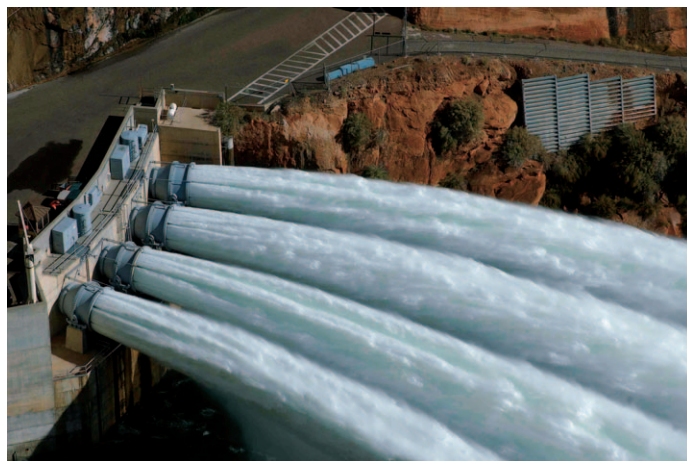
Figure 3. The Glen Canyon dam has altered water flow, sediment, and temperature regimes of the middle Colorado River for more than 40 years. Experimental releases of water have sought to reverse some of these environmental changes. For scale, the white grid lines at the top of the photograph are parking spaces. Photo: D. L. Blank.
